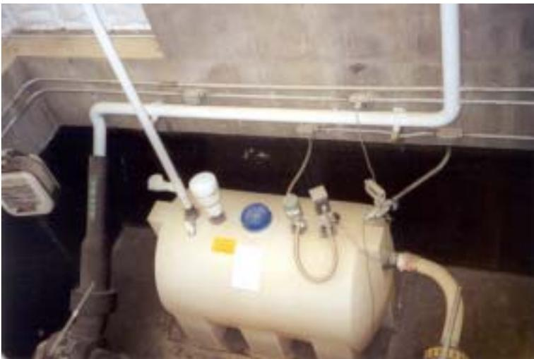
*Tank for the Leak Detection System in Valve House 1.*
